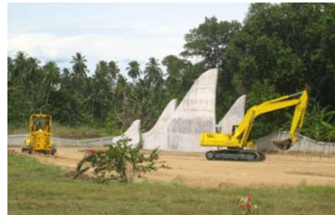
Workers constructing a tsunami memorial at one of the three mass grave sites in Banda Aceh. The remains of more than 4,000 people are believed to be buried here.
